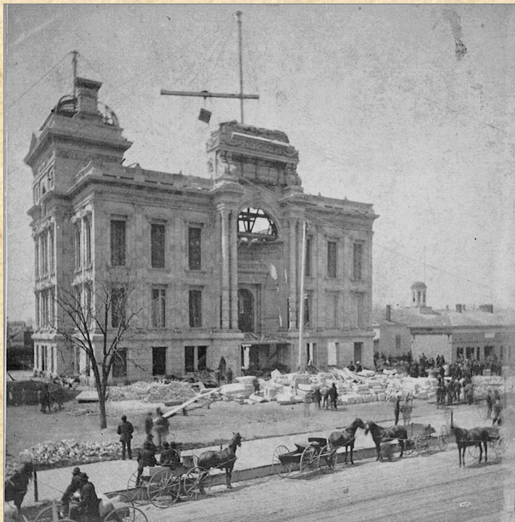
1877 photo taken of the courthouse after the collapse of the dome.
