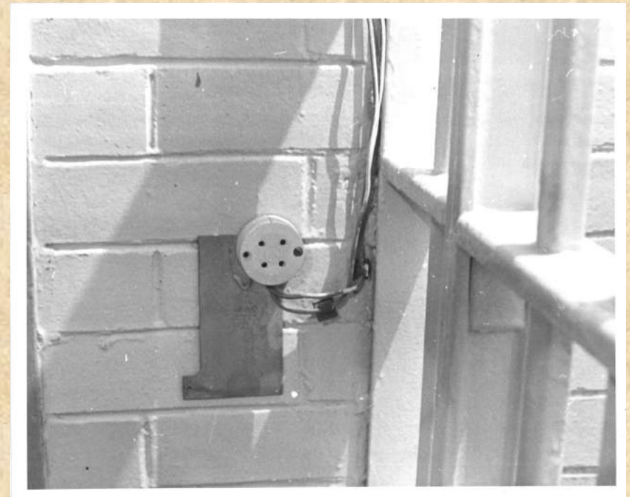
Back of photo reads: Phone jack that is located outside at the end of the cell-block. This is for security purposes due to the fact that it is not necessary to remove the prisoner from the cell-block when making a call.
